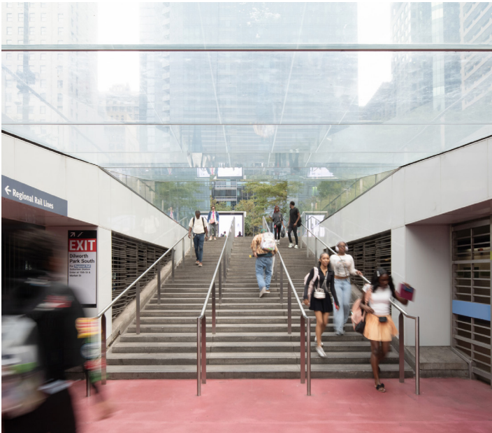
Headhouses bring light and protection from the elements to the SEPTA concourse below.
