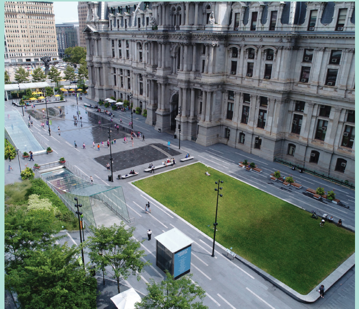
Dilworth Park glass headhouses (top, far left), fountain (top, center) and Albert M. Greenfield Lawn (bottom).
