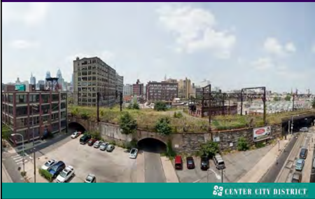
Masonry & stone retaining walls & earth fill
