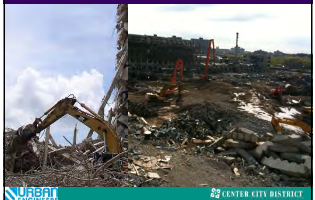
Urban Engineers: Full demolition: $120 million (2025) Includes $46 million removal/disposal of contaminated soil
