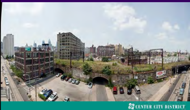
Created unsafe conditions in tunnels
