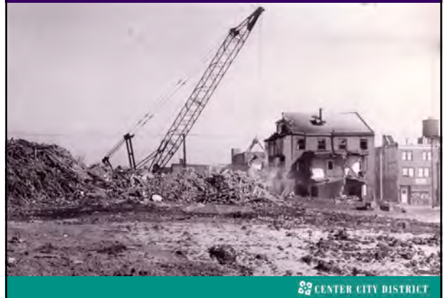
Demolition of hundreds of homes
