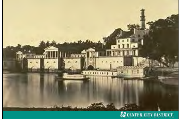
Pumped water from the Schuylkill River
