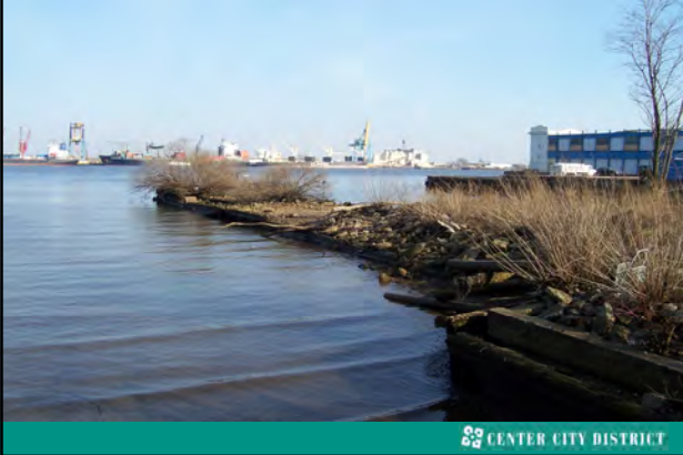
Left to deteriorate
