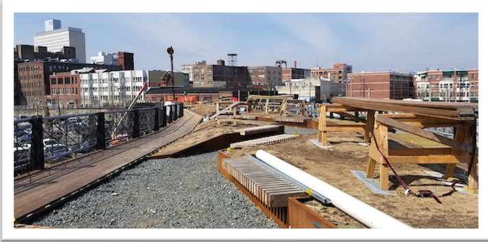
Figure 2 Phase I of The Rail Park under construction
