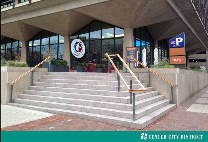
Stairs get built & La Colombe opens
