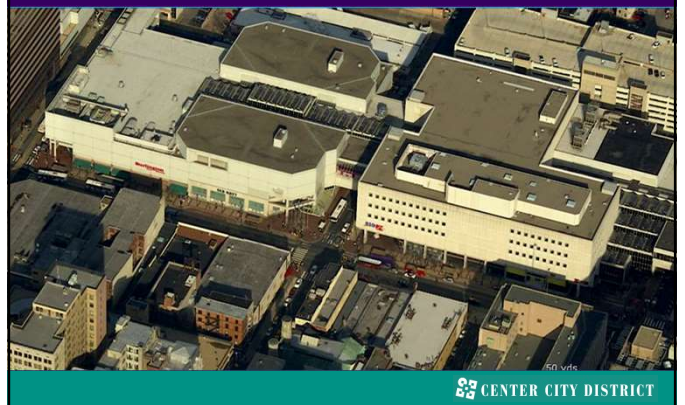
Largely inward facing orientation with a lot of blank walls
