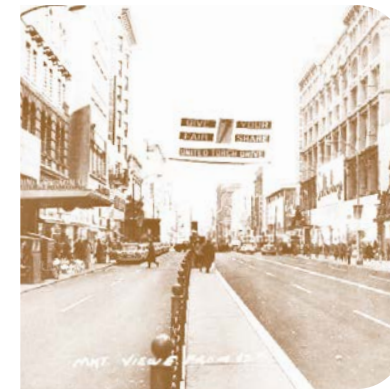
Market Street east from Twelfth Source: Center City District
