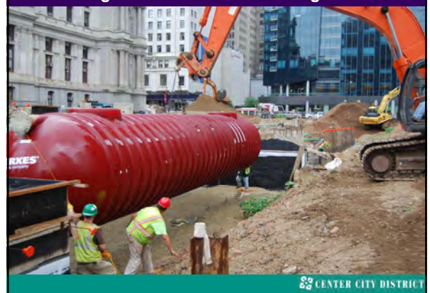
Storage tanks for installed during construction
