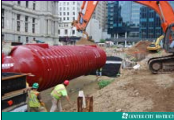
Storage tanks for installed during construction
