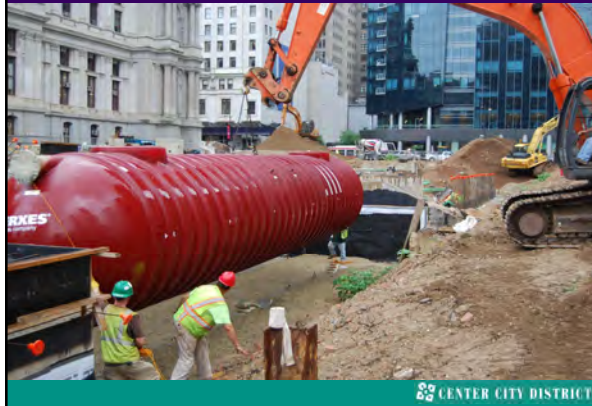
Storage tanks for installed during construction
