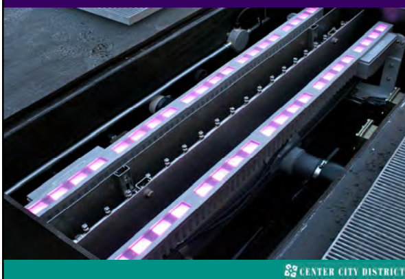
LED fixtures on either side of water jets
