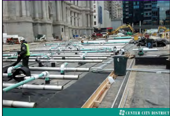
Plumbing & piping for fountain was installed
