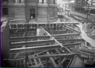
Subways & elevated lines followed: Broad Street line excavation under City Hall
