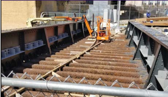
Ultimately, renovation: New brackets added to support new surface that was poured
