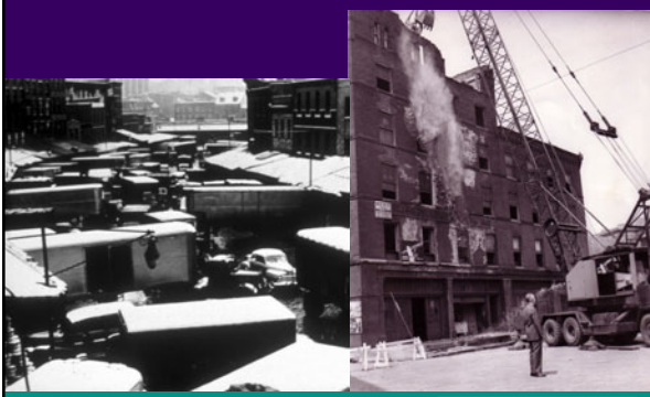
Dilworth supervises demolition
