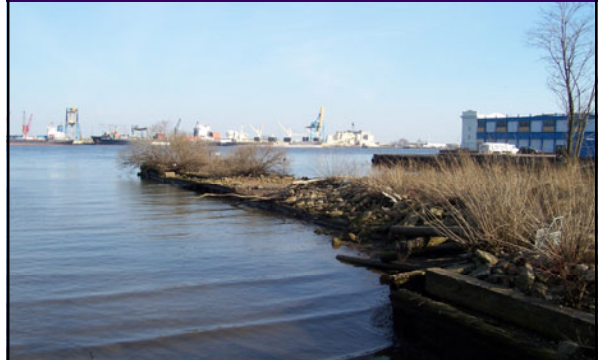
Left to deteriorate
