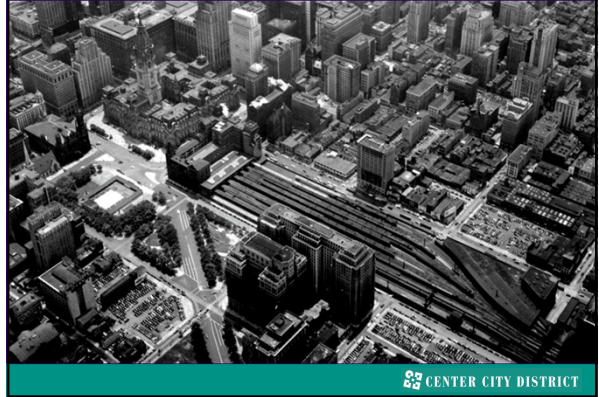
1953: the demolition of Pennsylvania Railroad
