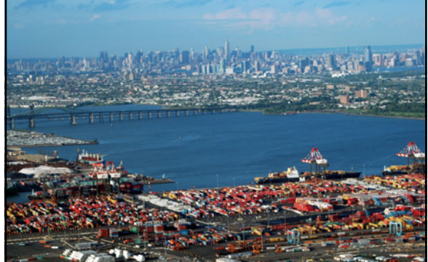
Port Elizabeth/Newark Marine Terminal
