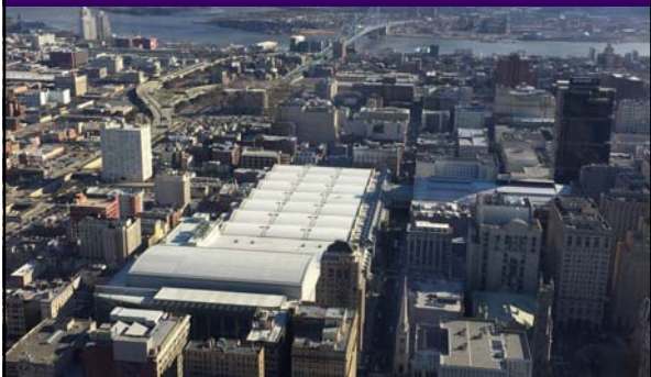
Convention Center under construction: Fear & opportunity
