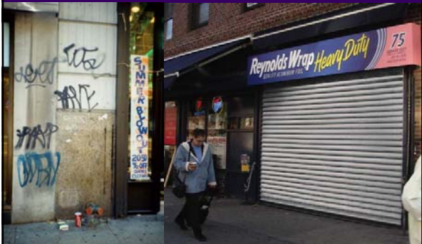
Neglected facades, solid security gates
