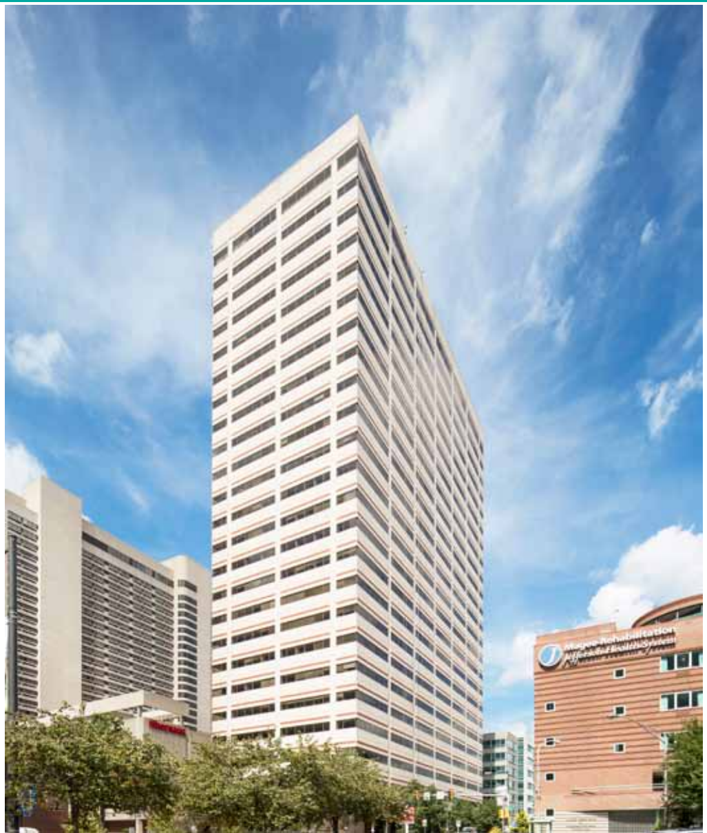
One Franklin Plaza is a recent example of a major office building whose prime tenant migrated elsewhere in the city, and the owner found insufficient office demand to replace it.
