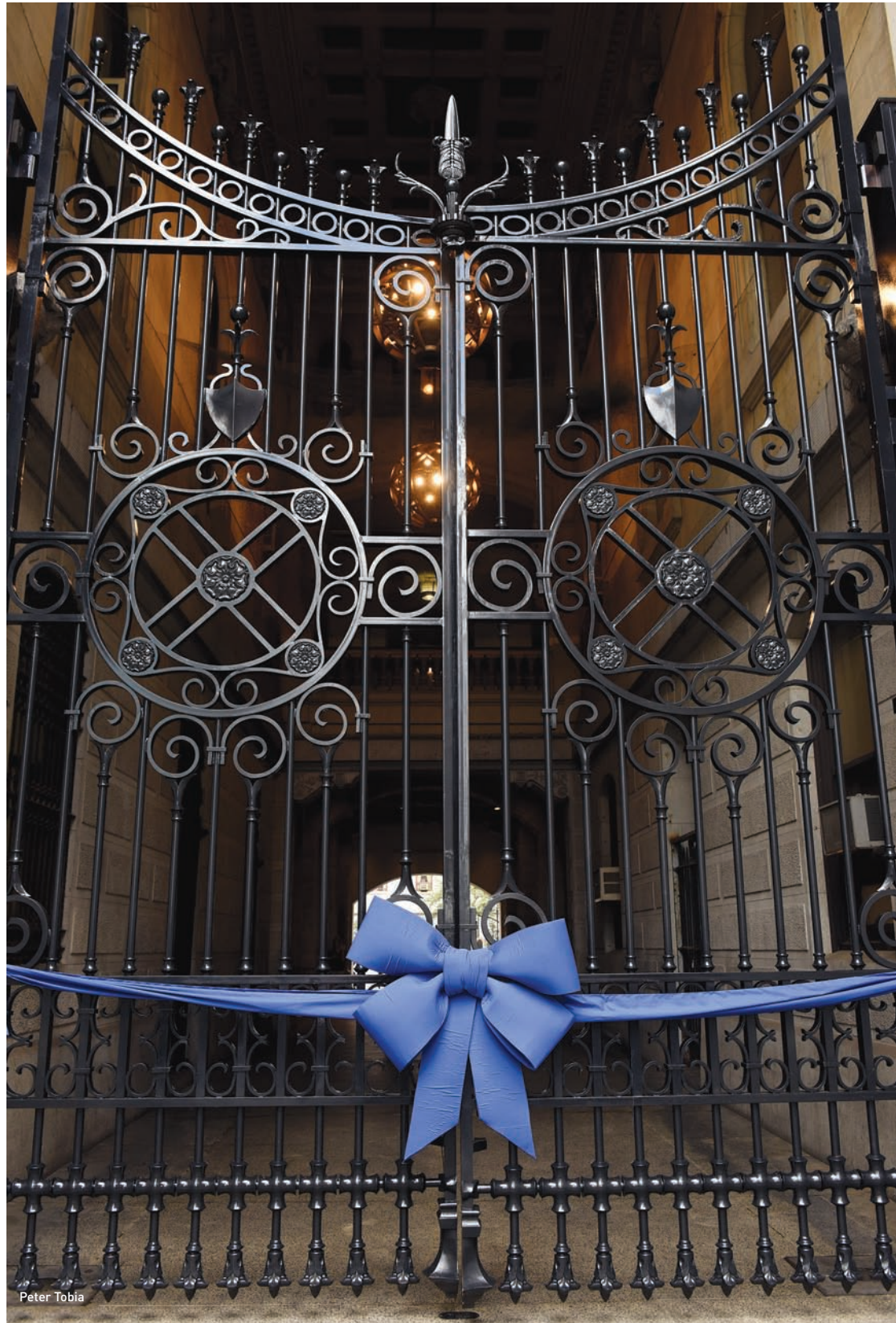
The gates are more than 25 feet tall and weigh approximately 3,200 pounds, even though they were forged using lighter weight stainless steel frames and aluminum castings.
