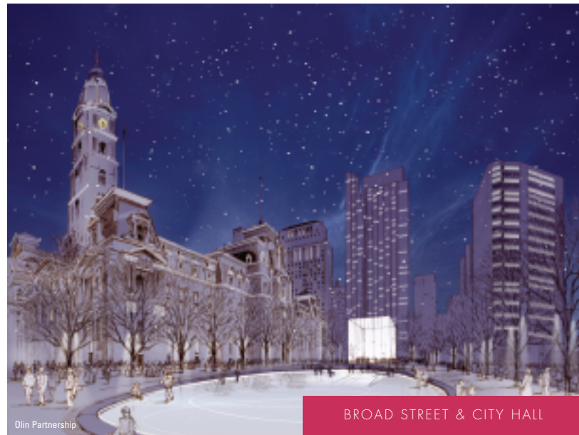
The west side of City Hall can become an animated civic space with a signature entrance to public transit, generous landscaping and a large fountain that can serve as a skating rink in winter months.
