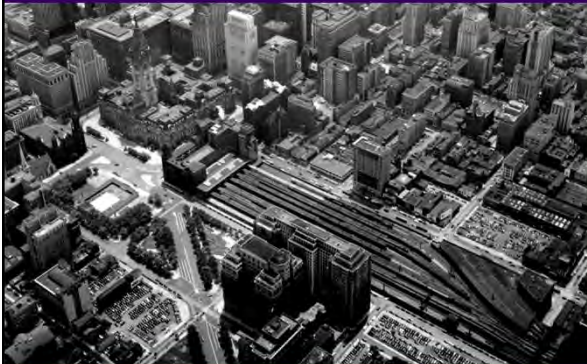
1953: the demolition of elevated railroad tracks
