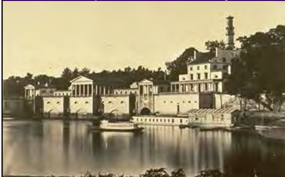
Pumped water from the Schuylkill River
