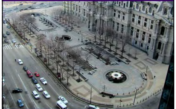
Barren 1970s failed space over transit lines
