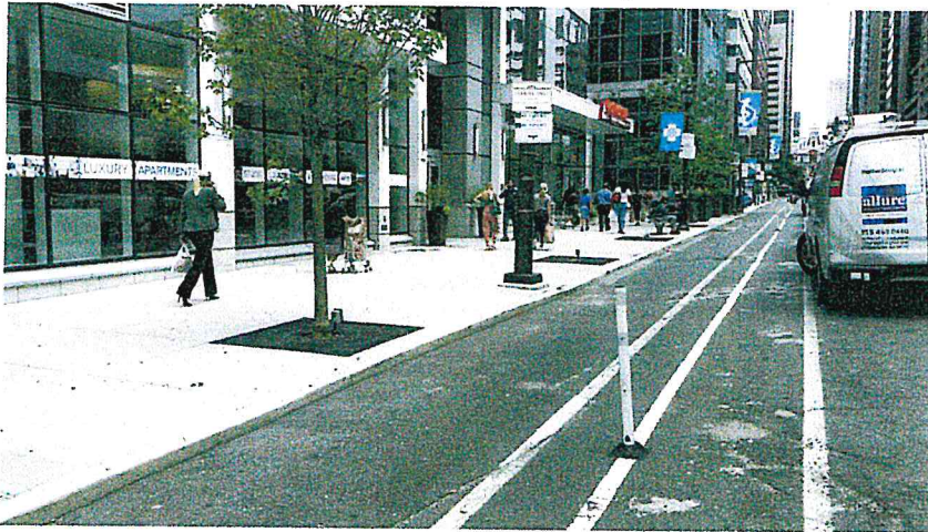
1900 BLOCK MARKET STREET VIEW B: EXISTING CONDITIONS
