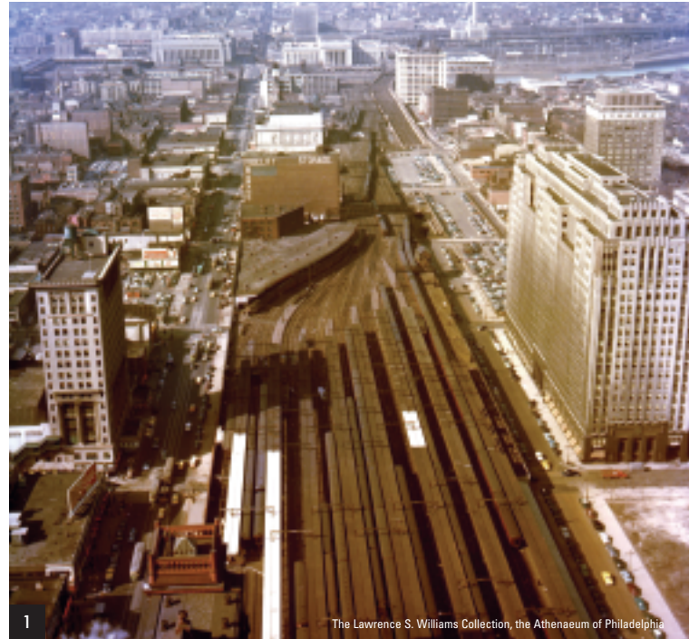
(1) View from City Hall: West Market and JFK Boulevard were created by a huge capital investment that placed rail lines underground and demolished the elevated tracks that formed a major barrier to development.
