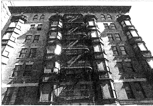
13th Street facade with fire escape
