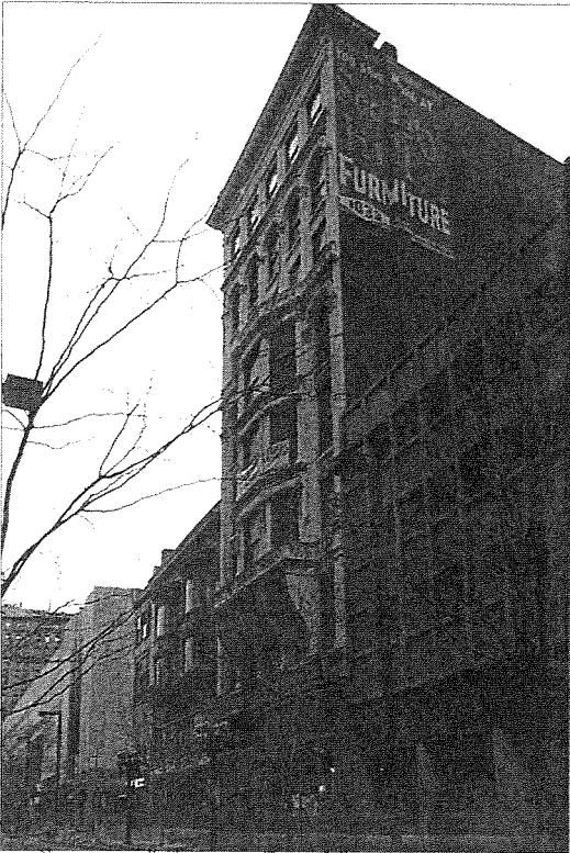
View to east showing adjacent vacant buildings
