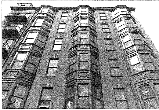
South-facing bay windows
